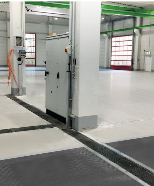
Production Workshop RULMECA in Aschersleben, Germany
