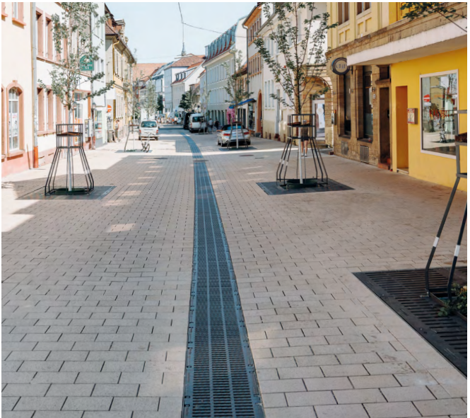
Rainwater treatment, tree irrigation with purified rainwater and discharge into surface waters in the city centre of Landau, Germany
